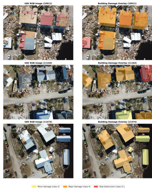
FIG. 1. Representative samples from RescueNet dataset: UAV RGB imagery (left) and corresponding building damage overlays (right) highlighting three damage classes directly on the imagery.
